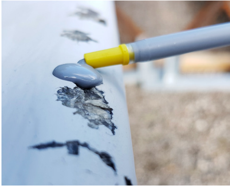
Erosion damages on a blade are studied using replication molding.
